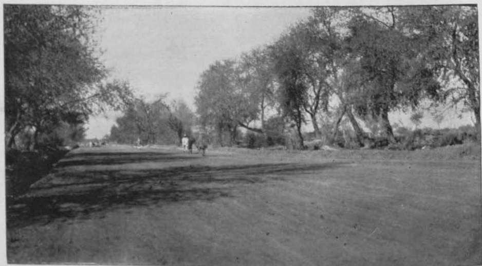
4. The finished road.
