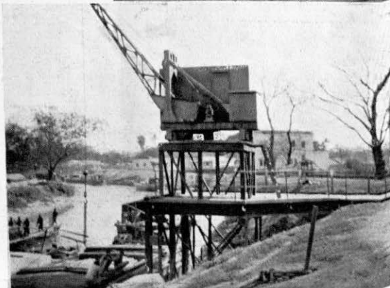
Gantry type:—Workers' contact with slewing cabin avoided by crane elevation.
